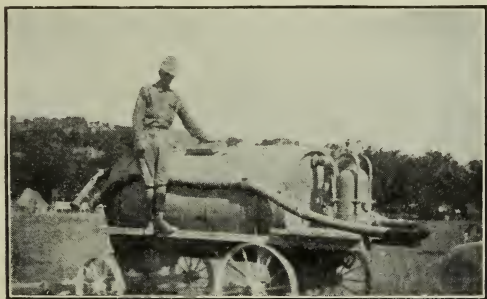
FIG. 45.—Excavator wagon and pump, best type. The wagon should carry the pump. Utilized to remove liquid waste from kitchens to septic tank.
